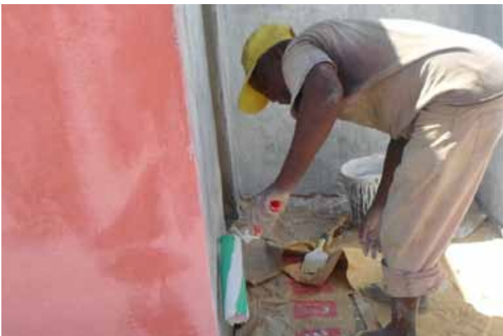
Construction of a school latrine.
