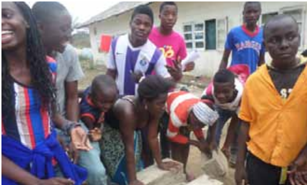
Water Assistants constructing latrines in the community, EPP Cabinda.
