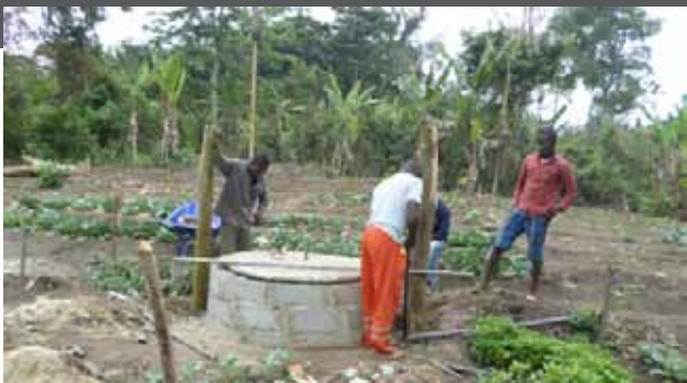
Installation of a Rope and Washer pump for irrigation, FC Bengo
