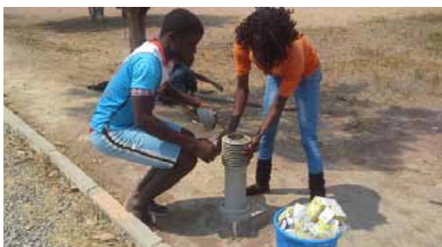
One of the girls demonstrating that girls too can work with electricity, EPP Kwanza Norte.
